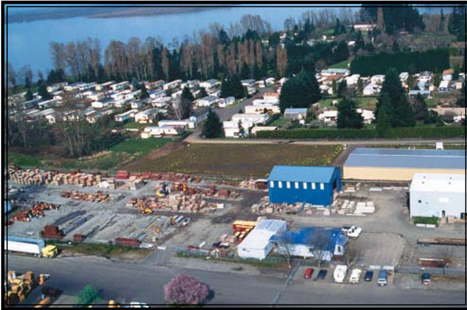
MASONS VANCOUVER , WA FORM YARD
